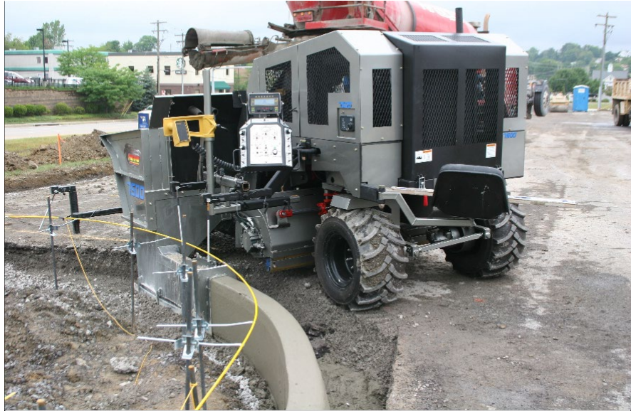
Accurate stringline setting for both straight and radius sections is a critical step in achieving the correct elevation of finished concrete.
