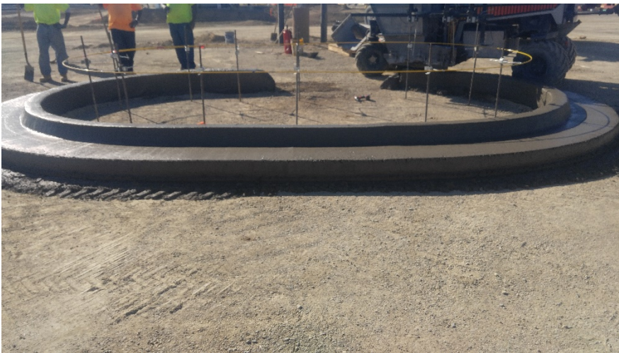
Figure 6. Fiberglass Radius-rod will require fewer stakes and increase radius precision.
